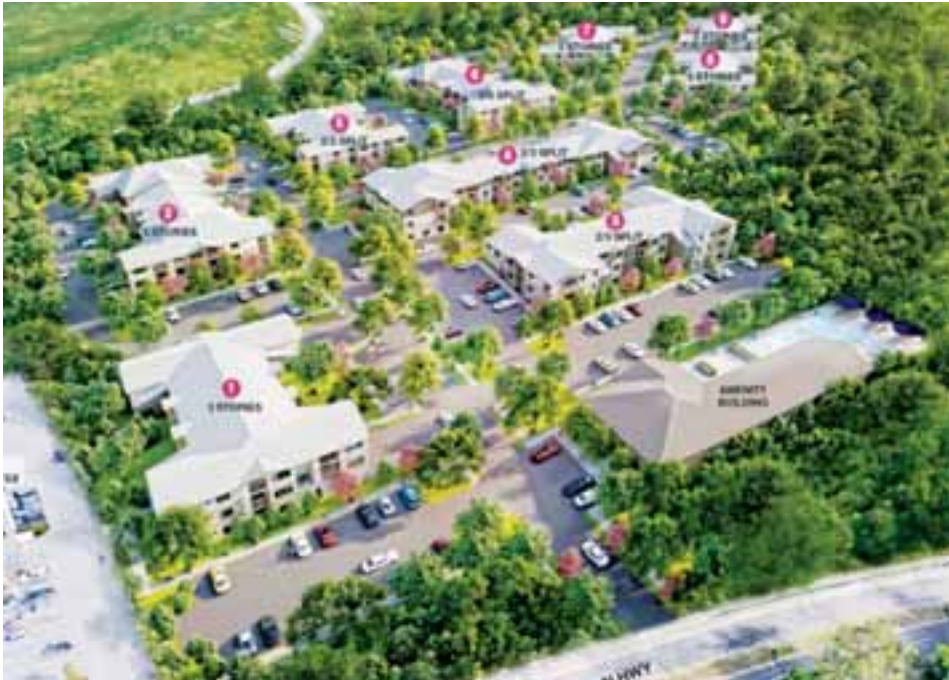
Residents expressed concerns with the tree canopy loss that would take place after this planned development for 990 American Legion Hwy. is completed.
