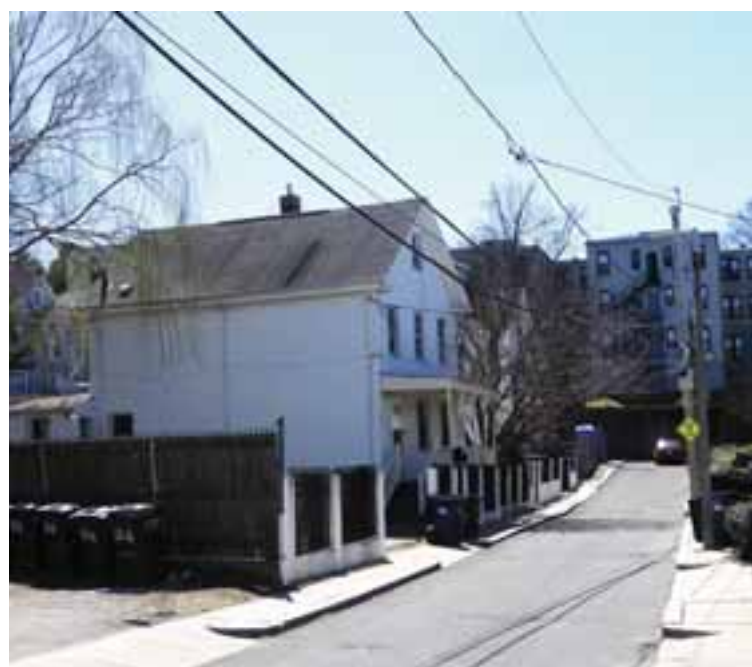
A look at the sites at 12 and 14 Ennis Road.
